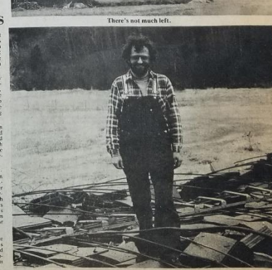
Demolition expert Carl Brandon surveys his handiwork.
